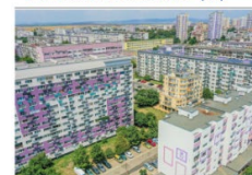
ENERGY TRANSITION OF CITY OF BURGAS (BG)
