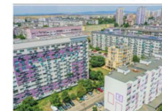
ENERGY TRANSITION OF CITY OF BURGAS (BG)
