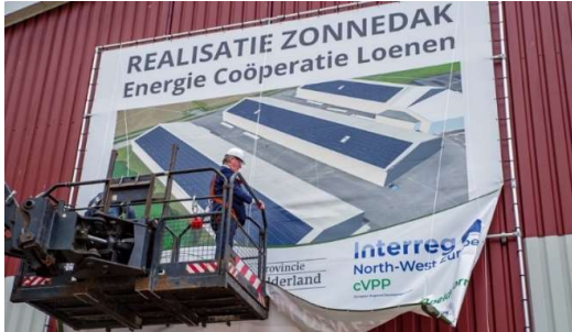
Figure 7: The first major project of Loenen Energy Cooperative 10
