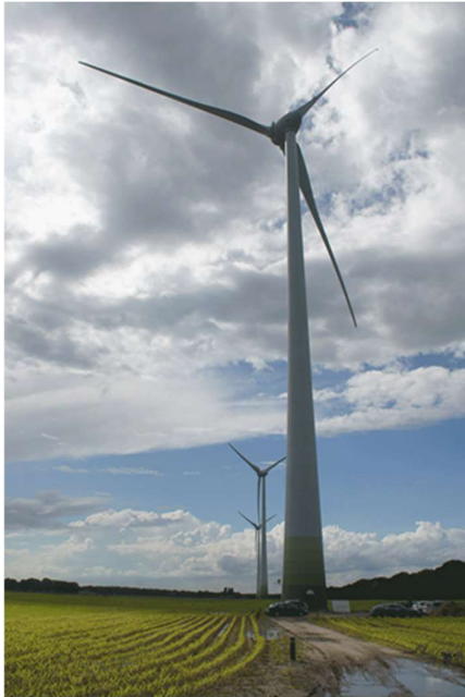
Figure 11: Weert Energy's wind park 18
