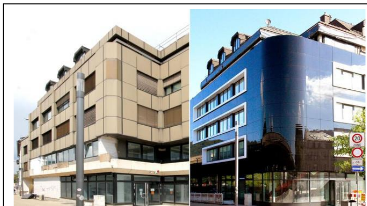
Before - After: The commercial building from the 1970s was almost completely covered with solar modules
